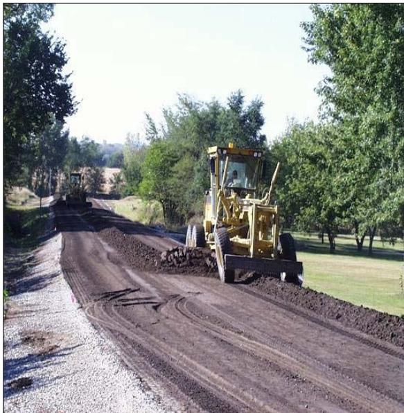
Full Depth Reclamation (FDR) is an effective recycling method for low-volume roads. Aged, worn-out roads can be rebuilt using the existing materials from the roadway. For FDR, generally fewer materials are needed and hence fewer trucks are needed to transport the materials. FDR is also considered environmentally friendly because it decreases the amount of materials entering a landfill.
